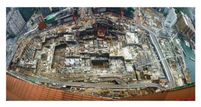
Deep excavations in urban areas need to limit ground movements for the protection of surrounding property and generally have limited space for construction. Top-down construction addresses both issues. Lateral earth support is provided by progressively excavating and constructing permanent robust supporting structures and the completed decks provide working space.
