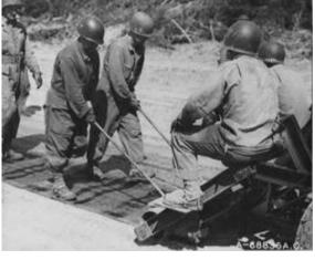
monsoon season. In northern France and Belgium in 1944/45 they allowed rapid surfacing of temporary or expedient airfields by sealing the ground and maintaining the existing soil's bearing capacity, thereby enabling close tactical air support to be maintained with rapidly advancing ground forces. They are currently under consideration for rapid repairs of airfield crater damage.
