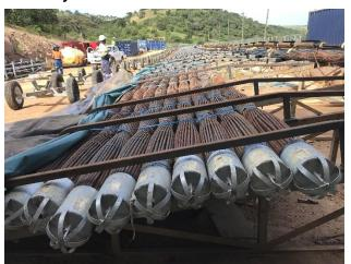
Grouted anchors are a technology that is extensively used on a worldwide basis for the support of geotechnical engineering structures. These can vary from retaining structures for slopes and deep excavations, applications for uplift resistance in tunnels and storage tanks with working loads typically up to 2000 kN, to ultra-high capacity systems used for dam upgrades with test loads exceeding 19000 kN.
