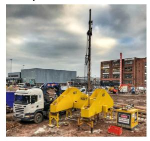
In 2018 the ICE released the 3rd edition of the Specification for Piles and Embedded Retaining Walls (SPERW). Acceptance criteria for static pile testing has now changed to improve quality and safety.
