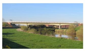
Newland Bridge is a 3-span steel composite structure carrying the A645 over the River Aire between Drax and Goole.
