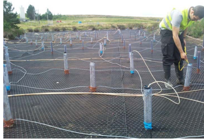
Electrodes installed by hand
