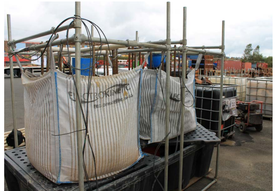
Solidification of drilling mud
